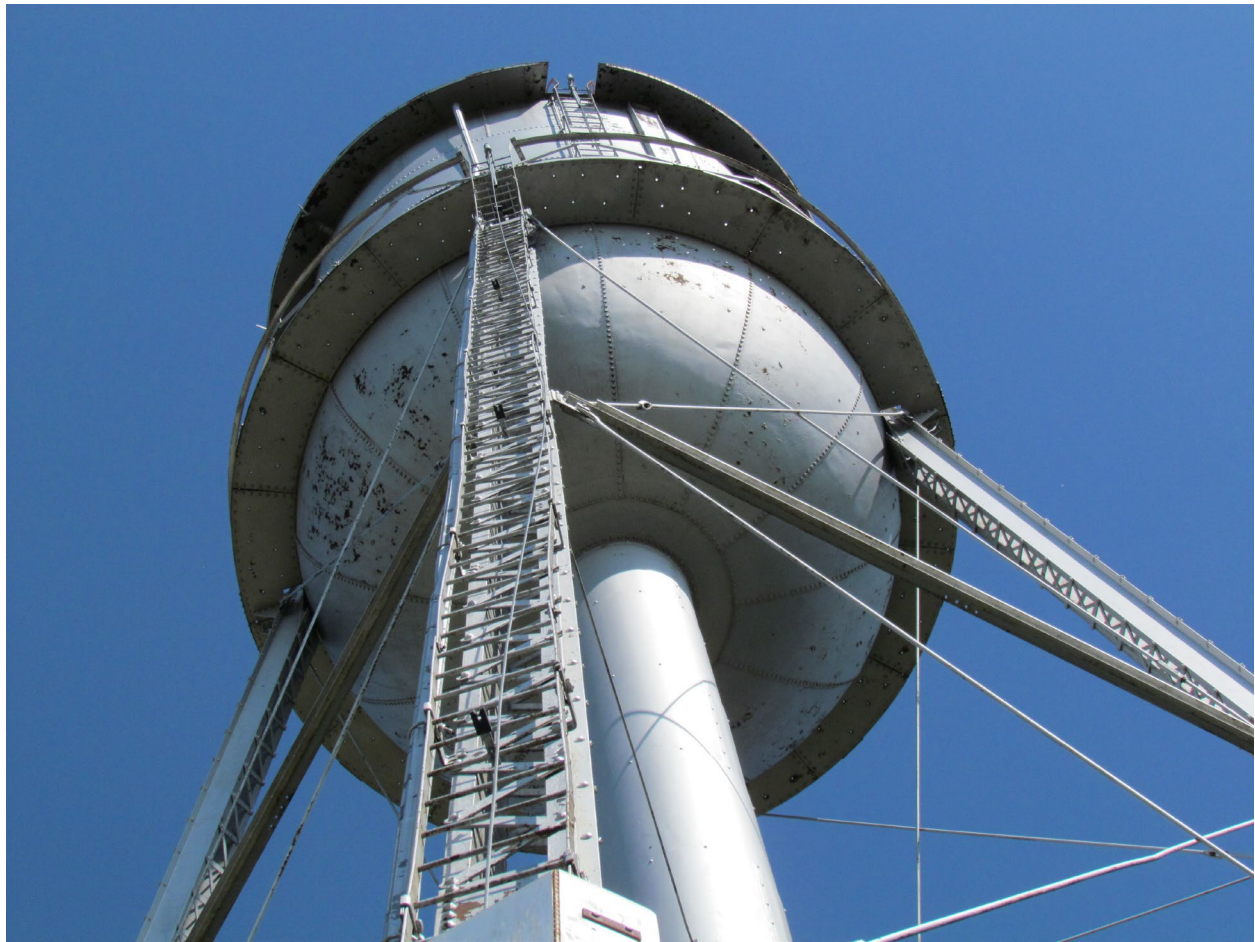
Figure 10. View up northwest leg of Essex Water Tower (site 73-00180), facing southeast, showing built-in ladder and raised tank.
