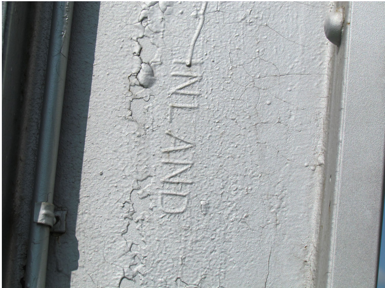
Figure 9. Detail of "INLAND" stamp on steel I-beam in northwest leg of Essex Water Tower (site 73-00180), facing northeast.
