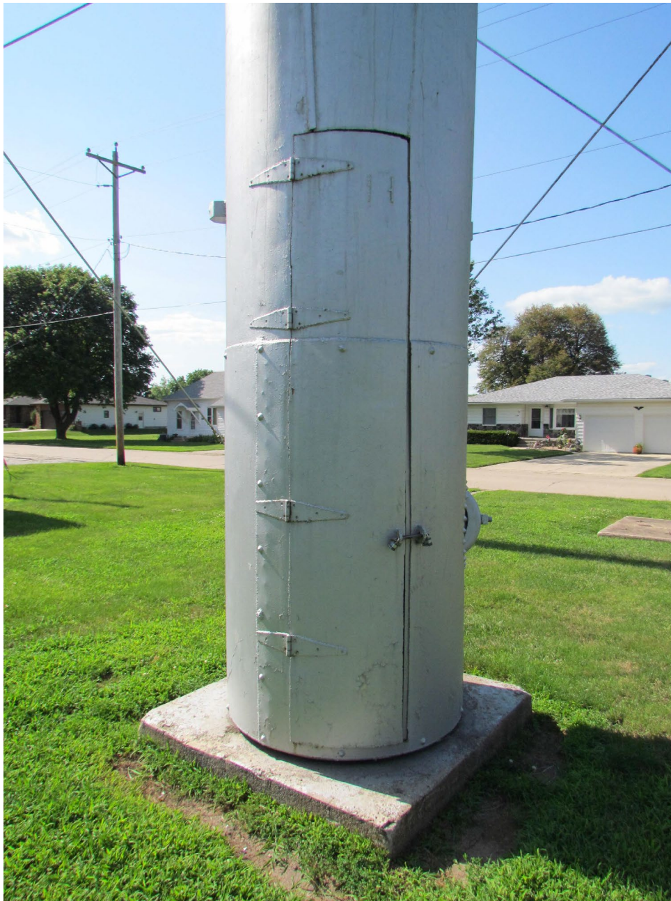
Figure 8. Detail of hinged opening at base of frost jacket of riser pipe on Essex Water Tower (site 73-00180), facing northwest.
