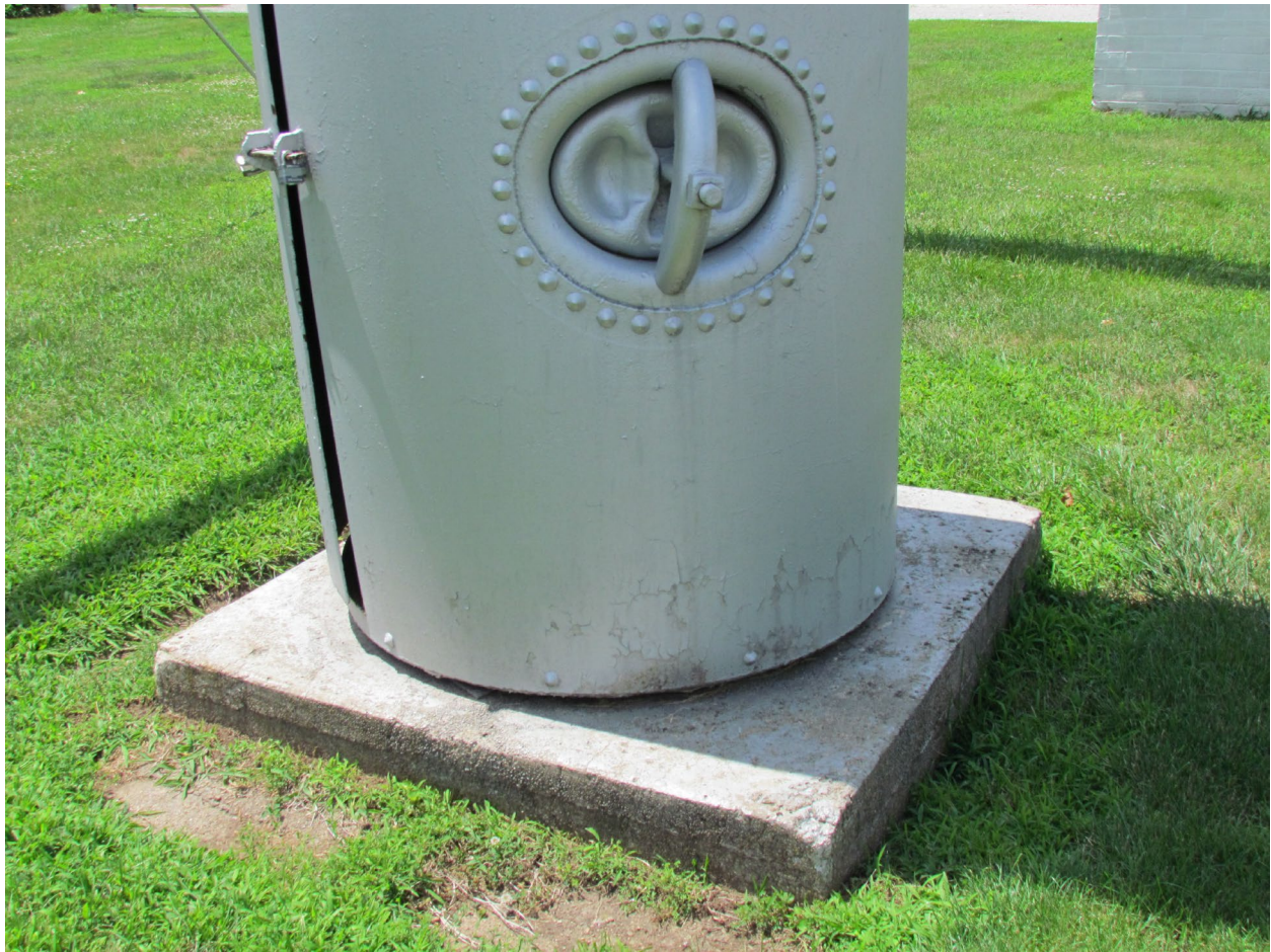
Figure 7. Detail of inspection cover at base of frost jacket of riser pipe on Essex Water Tower (site 73-00180), facing southwest.
