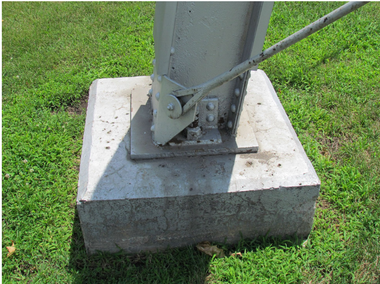
Figure 6. Detail of concrete pier under northeast leg of Essex Water Tower (site 73-00180), facing south-southwest. The small cross in the north east corner (indicated by an arrow) is evidently a bench mark elevation to establish centerline grades of streets in Essex; see Public Notice: Town of Essex, Iowa, Ordinance No. 91, The Essex Independent, November 21, 1968, p. 8.
